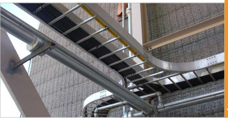
ly used to implement intelligent systems. Selecting inappropriate brackets dramatically reduces system performance. Also, the type and the material of such support equipment are different based on their use and performance in different places. Implementing ladders in buildings as well as connecting racks to each other in data centers is also very important considering the size of cables.
