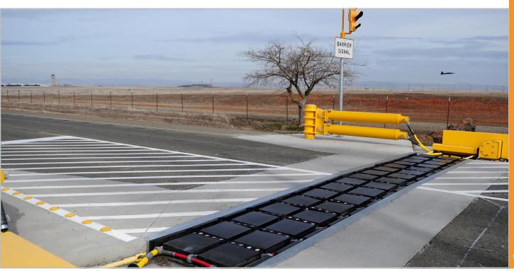
with smart card readers or cashon-access points make it possible for people to cross. Vehicles' gateways are usually used to authenticate drivers and passengers. However, barrier gates do not have high protection, but the security bollards prevent any penetration. Various video equipment for checking the under part of the vehicle is also installed on this system.
